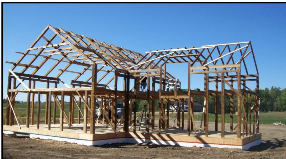
Modified and Re-Installed
