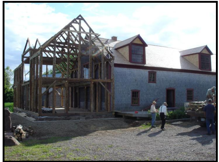
Original 1795 Summer Kitchen Cape
