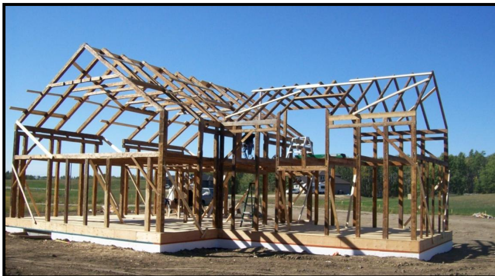
Modified and Re-Installed
